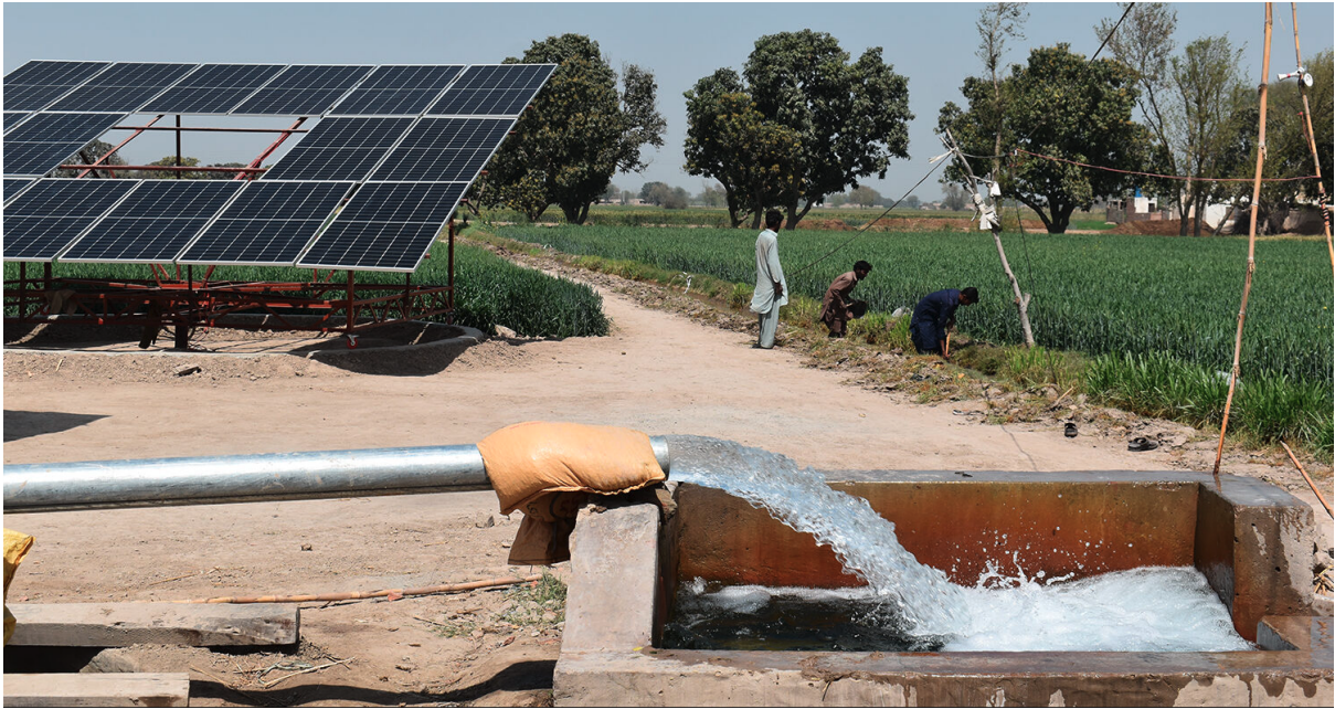
Solar powered tube wells in Pakistan. Credit: CGIAR
